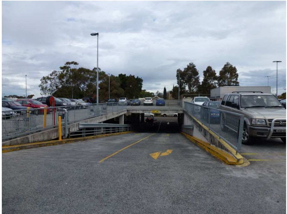
Figure 4 – View from roof top carpark
